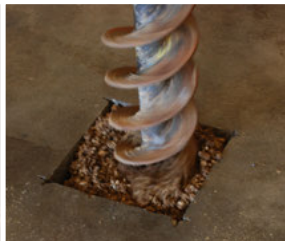
Auger hole for cylinder.
