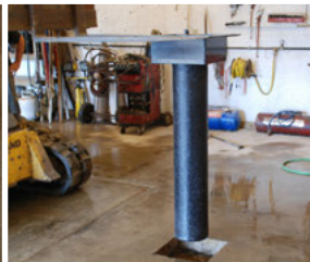
Place cylinder in hole.
