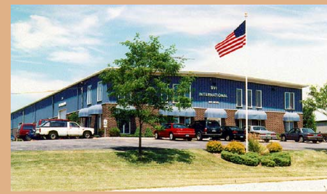
Main office and warehouse facility
